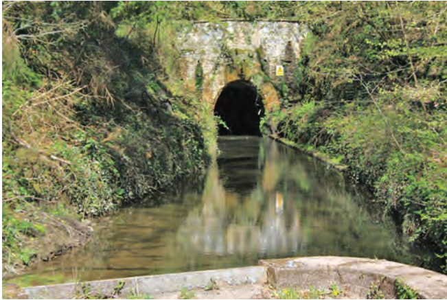
Southern portal of the tunnel
